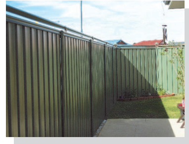
Oscillot™ as installed along a very satisfied Perth customer's fenceline
